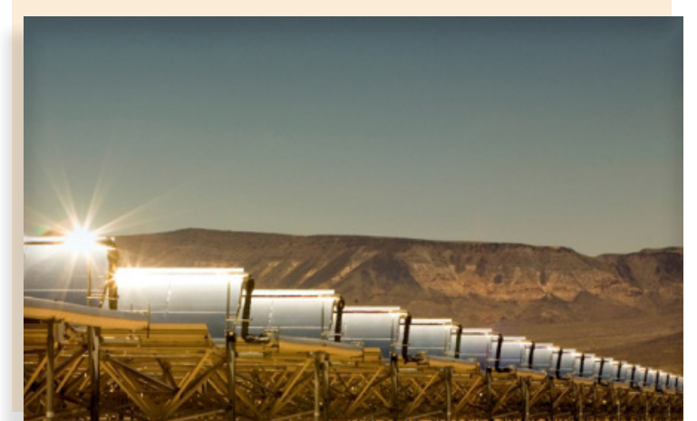
Solar farm located in the valley.
